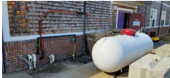
Propane tank located outside of original Mech room which feeds new instantaneous propane fired domestic water heaters.
