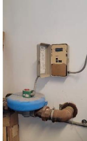
Single Propane tank to feed Gas turrets in Science classrooms, along with a main gas shut off.
