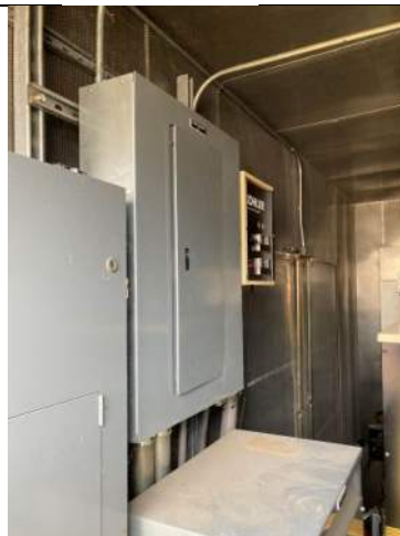
Automatic Transfer Switch
