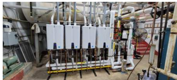
Main (4) Boilers in 1959 Mechanical room (4) Instantaneous water heaters with 1,000 Gallon Storage tank behind
