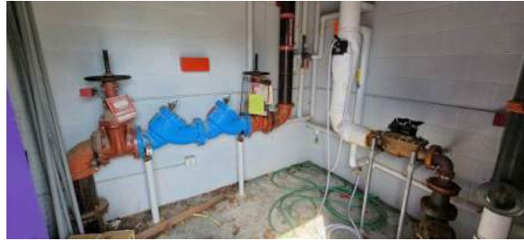
6" Service in portion of building constructed in 1990s
