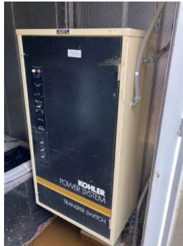
Automatic Transfer Switch
