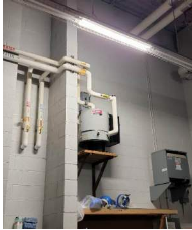
Small Electric water heater feeding Custodial area near 1990s Mechanical room
