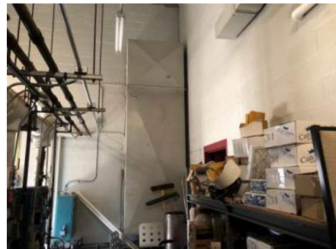
Combustion Air Intake
