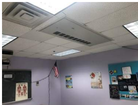
Ceiling Classroom Unit Ventilators
