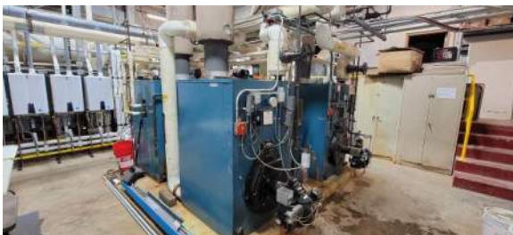
Main (4) Boilers in 1959 Mechanical room (4) Instantaneous water heaters with 1,000 Gallon Storage tank behind
