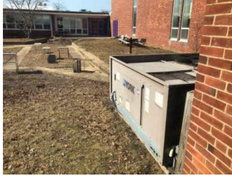
Outdoor Air-Cooled Condenser
