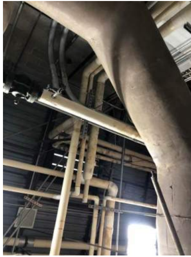
Combustion Air Intake
