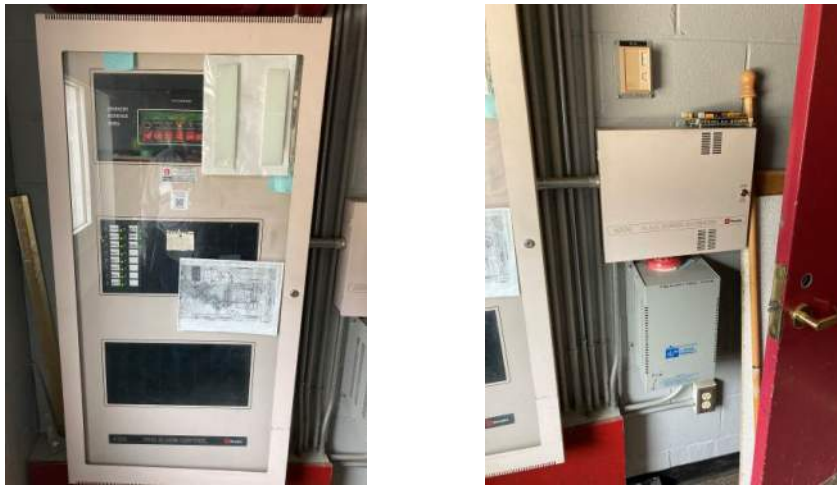
Fire Alarm Control Panel and Notification Device
