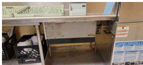
Electric booster heater
