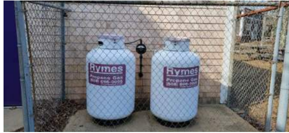
(2) Propane tanks to feed kitchen equipment for Culinary kitchen.
