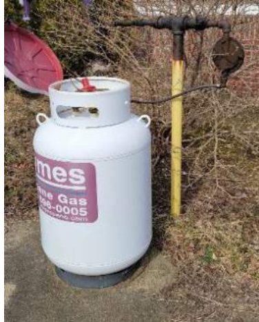
Single Propane tank to feed Gas turrets in Science classrooms, along with a main gas shut off.
