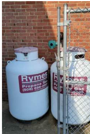
(2) Propane tanks to feed kitchen equipment for Main kitchen.
