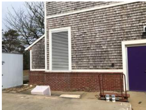
Combustion Air Intake
